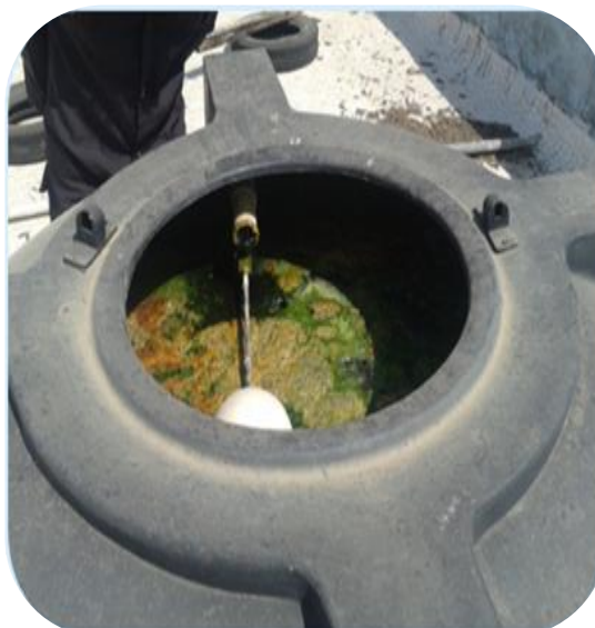
Poorly Maintained Water tank with Algae- SDH Khedbrahma, Sabarkantha
