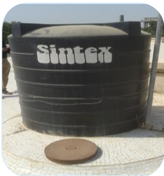
Open Overhead tank with cover near it – CHC Naliya, Kutch,
